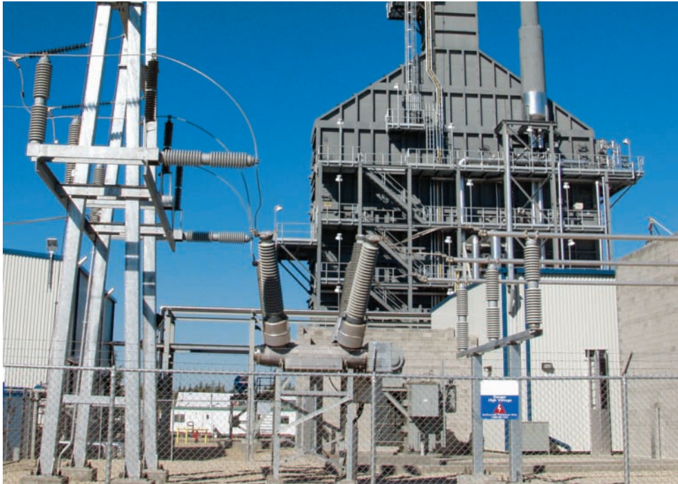
TransCanada's Bear Creek Cogeneration Plant uses natural gas and wood waste to generate electricity and steam.
