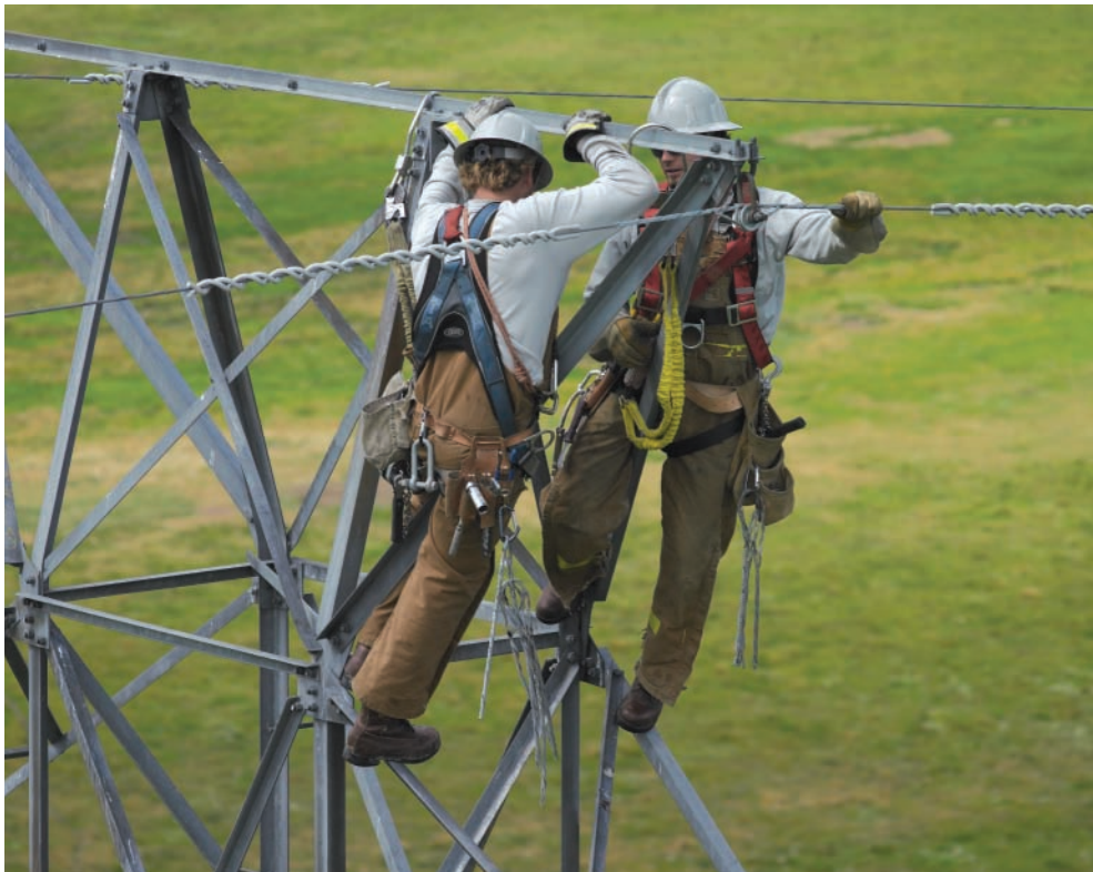
Upgrading overhead shield on a transmission line west of Edmonton.
