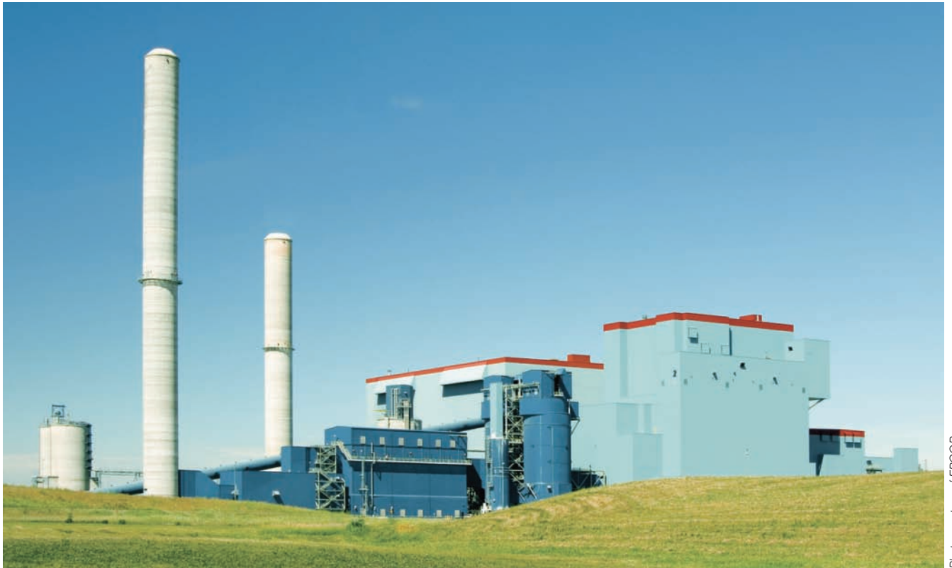
EPCOR Genesee Generating Station with the addition at left of Unit 3.
