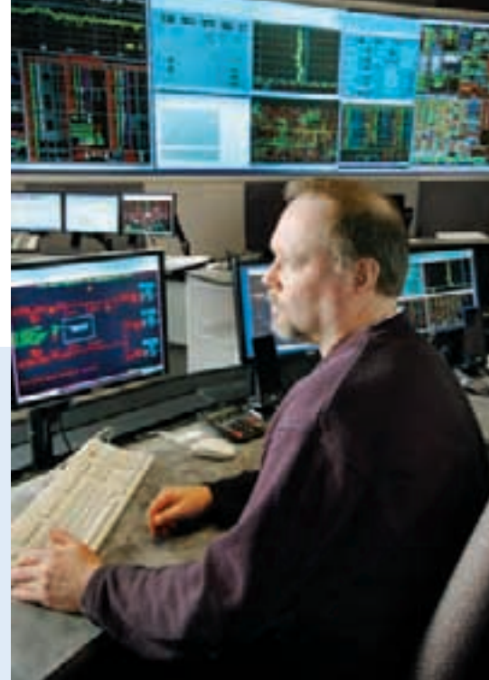
An AESO system controller monitoring Alberta's power grid.
