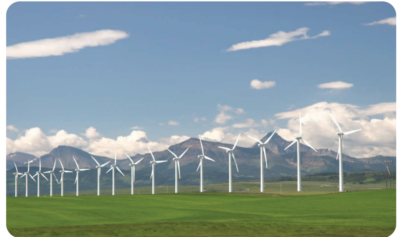
Alberta's wind industry has dedicated valuable time and resources to wind development during the last few years. The AESO will continue working with our stakeholders to manage the future potential of wind development in Alberta.
