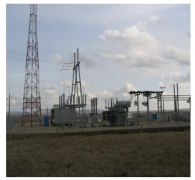
The proposed substation site will be 60 metres x 60 metres (197 feet) in size and will include associated equipment, such as a transformer, that reduces the voltage of electricity carried on the transmission system. It will also include a 25 metre high telecommunications tower. The substation site will be surrounded by a chain link fence and accessible through a locked gate by authorized personel only. It will be similar to the substation pictured to the left.
