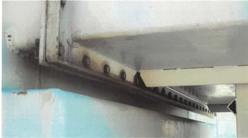
Figure 5 Kennedale Tx1 - Sweating flange between main tank and LTC compartment
