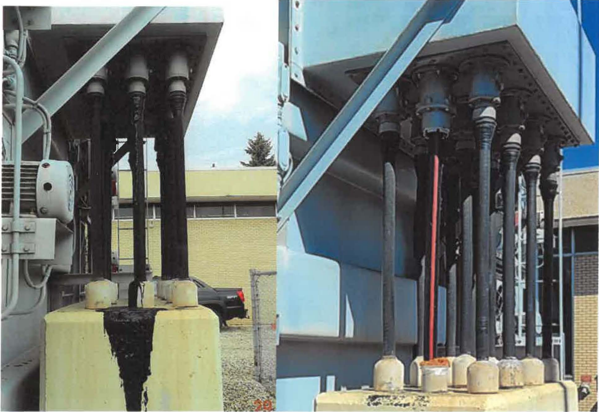
Figure 8 Kennedale Tx2 - Failed secondary cable connection and the retrofit solution
