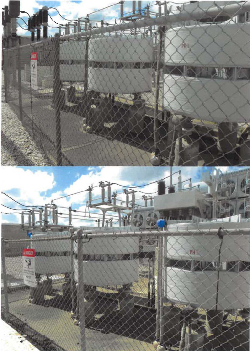
Figure 9 Kennedale Tx1 (Top) and Tx2 (Bottom) Dry Type Reactors
