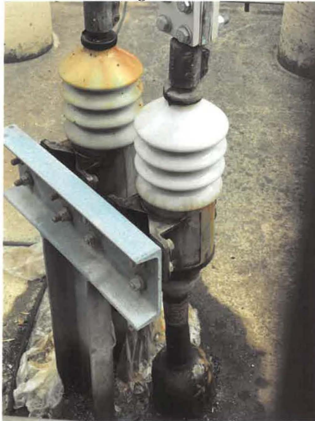
Figure 11 Leaking PILC Cables
