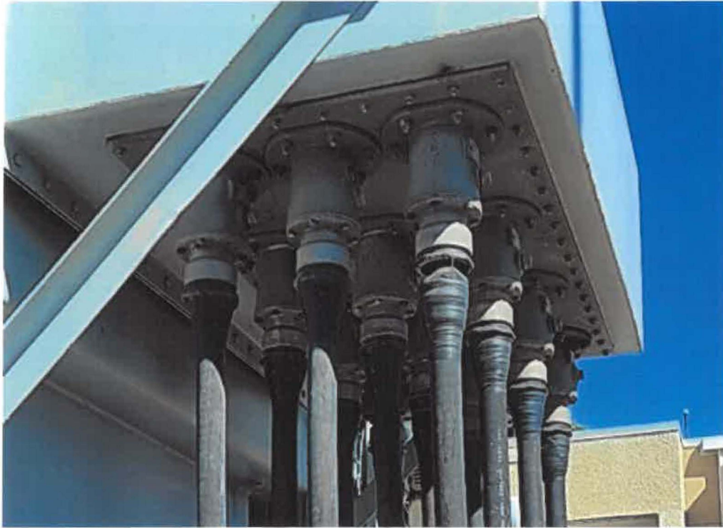
Figure 6 Kennedale Tx1 - MV cables
