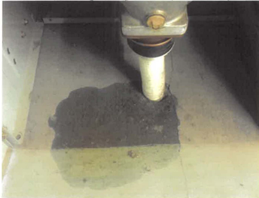
Figure 10 Leaking Switchgear Cable (outside of cell)
