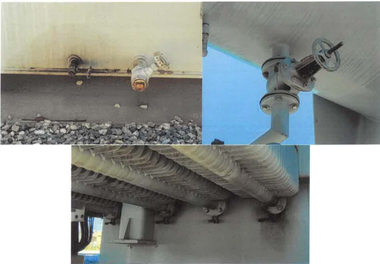
Figure 7 Kennedale Tx2 - Minor sweating from valves
