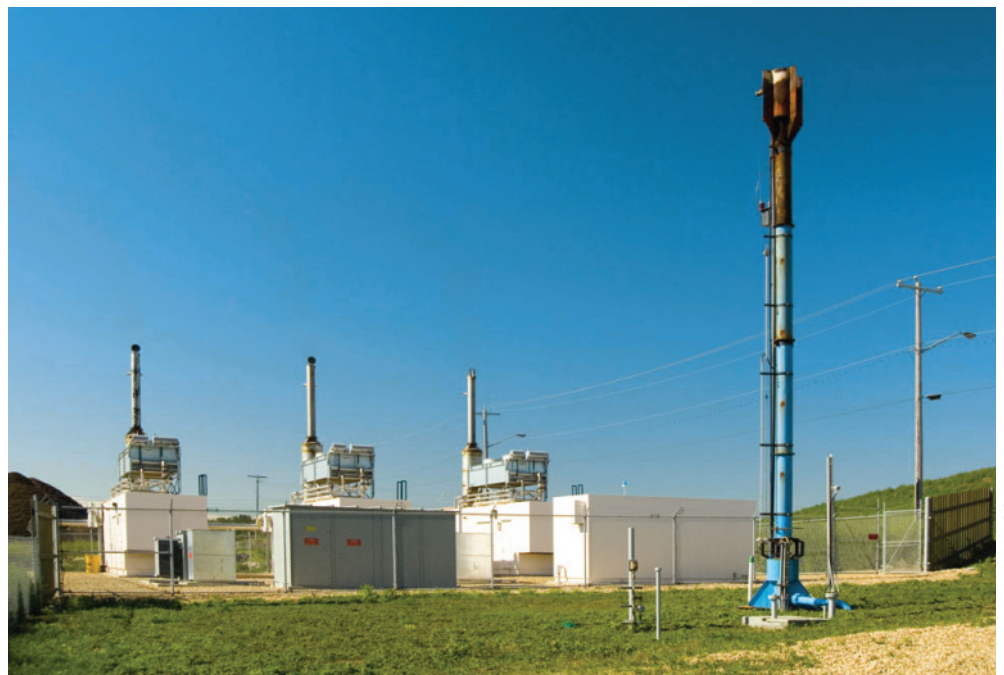
EPCOR's 4.8 MW Clover Bar landfill gas facility in Edmonton is the first of its kind in Alberta to both recover methane and use it to generate electricity.
