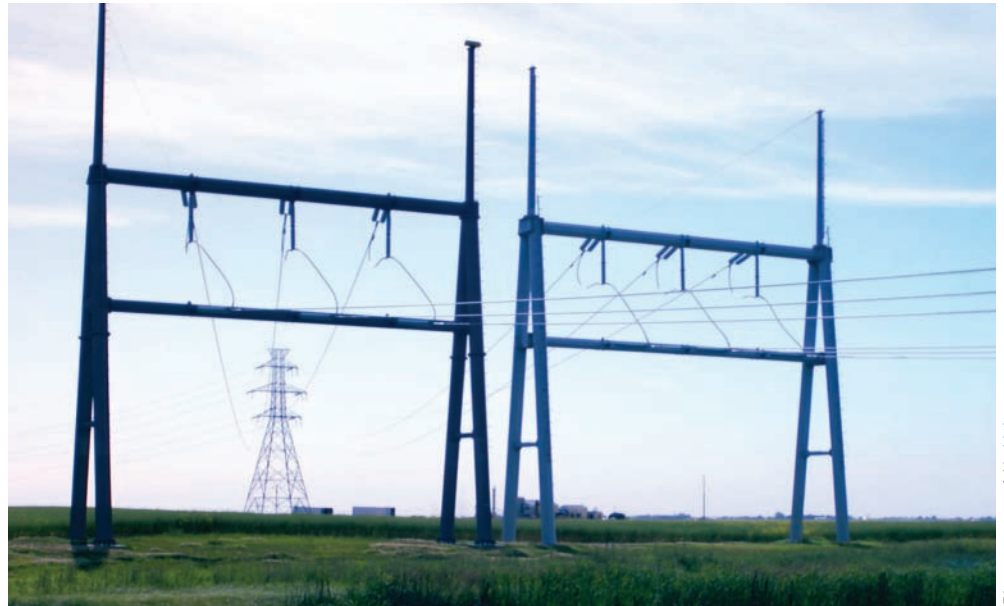
A-frame structures at the Langdon substation east of Calgary.
