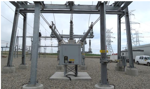
A typical 138 kV circuit breaker is pictured above.
