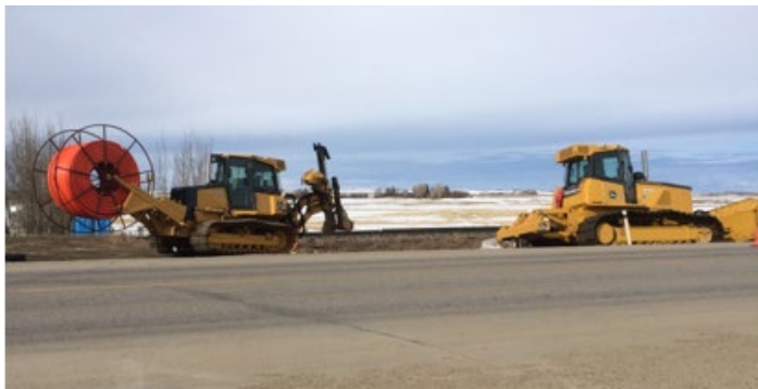
Above: Fibre optic cable being buried. You may see similar construction activities in your area.
