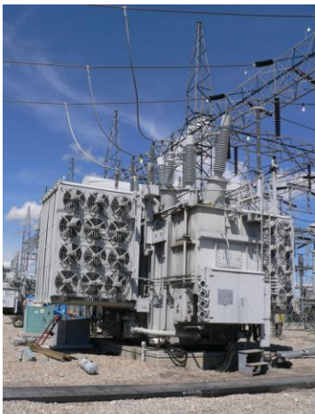
Above: example of a 138/25 kV transformer
