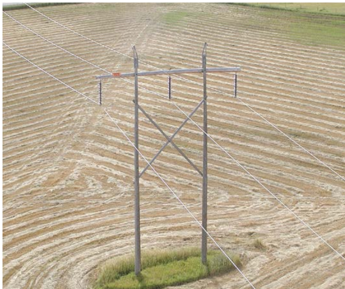
The structures on the proposed 1181L line will look mostly similar to the above, but the insulators may be configured differently.
