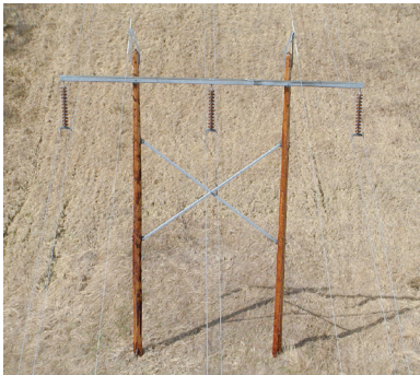
A typical single-circuit 240 kV wooden H-frame structure
