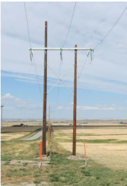
Above: A typical two-pole wood structure.
