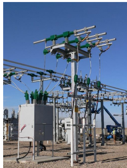
A typical 25 kV circuit breaker is pictured above.
