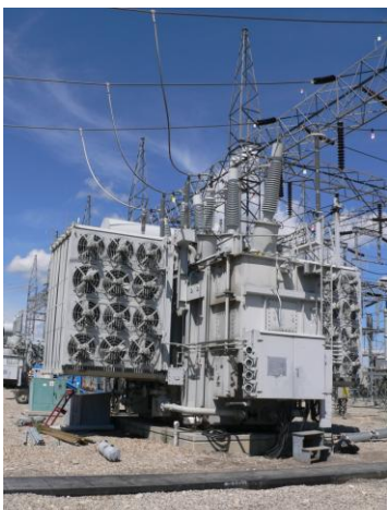
Above: example of a 138/25 kV transformer
